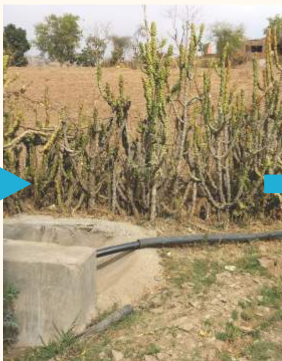
A pipeline connected to an underground well helps in supplying water to tank situated at an elevated level in Udaipur
