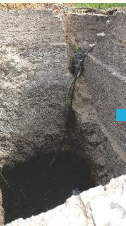
A pipeline connected to an underground well helps in supplying water to tank situated at an elevated level in Udaipur
